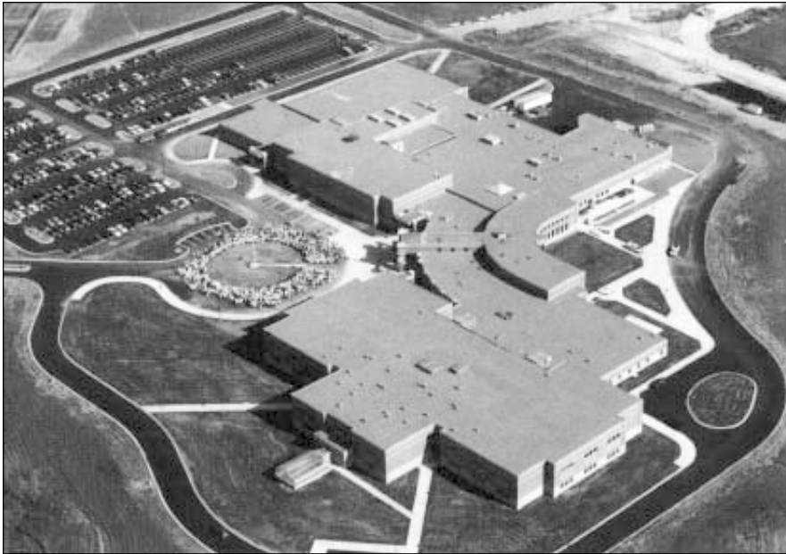
The new 267,000-sq-ft Red Wing High School benefits from six energy recovery units, quiet fans, round ductwork, and efficient boilers and chillers while retaining the ASHRAE ventilation requirements and saving more than $400,000 in first costs.
