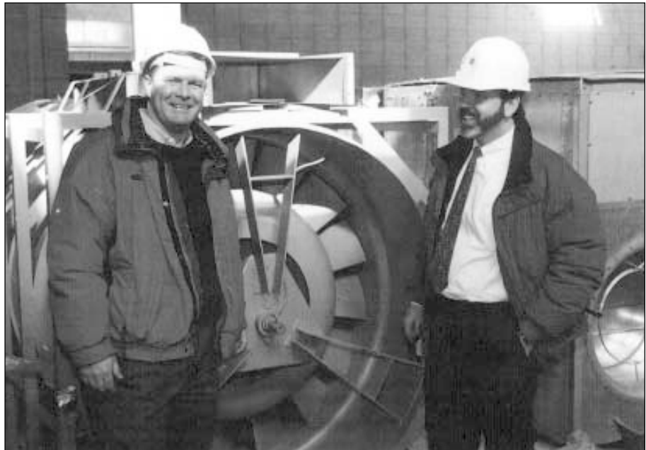
Tom Bredesen, of The Trane Company, and John Brady, of Armstrong, Torseth, Skold, and Rydeen Architects and Engineers, on the job at the Red Wing High School.
