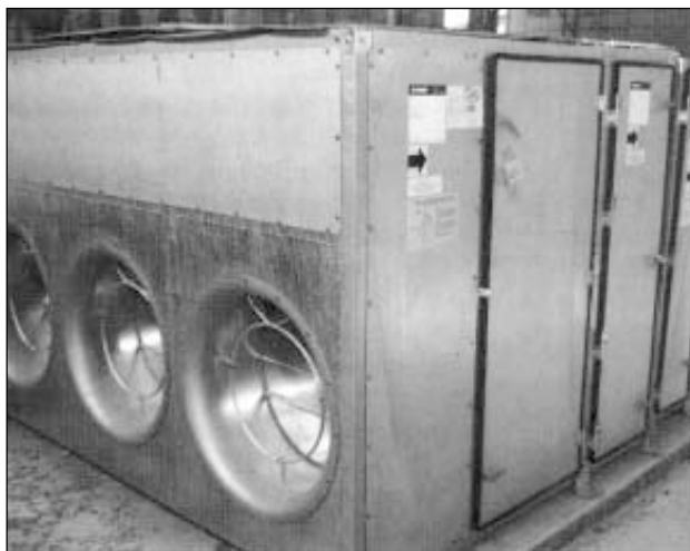
Trane Company ‘Modular Climate Changer’ air handlers with integral ‘Traq’ dampers to meter outdoor ventilation air.
