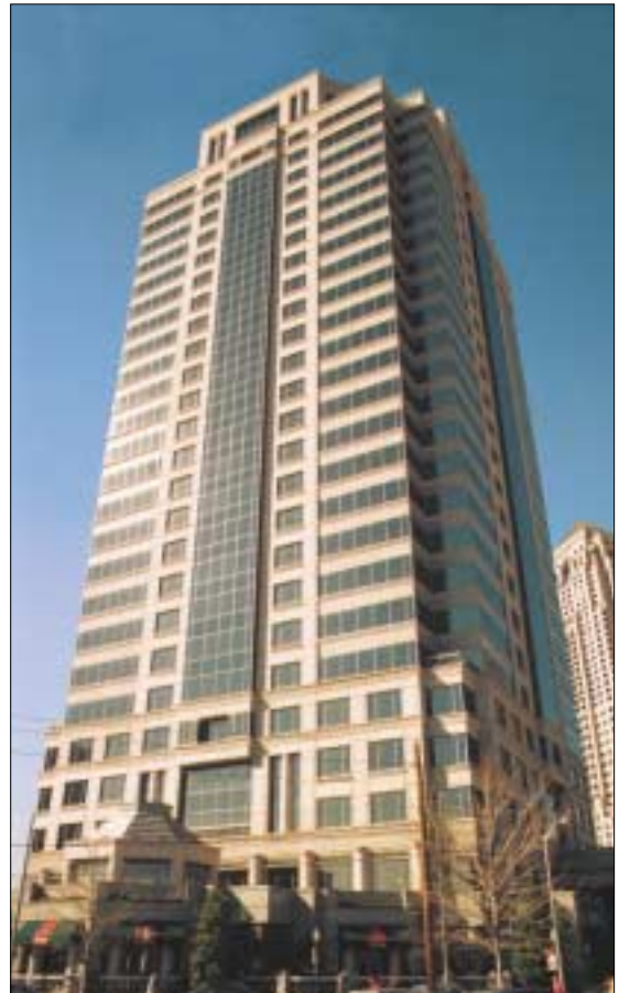
The desiccant-based energy recovery system at Eleven Hundred Peachtree Street pre-conditions ventilation air by removing the moisture before it enters the air handlers.
