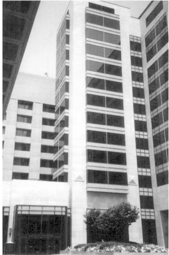
Johns Hopkins chose a desiccant-based system for its Ross Research facility.
