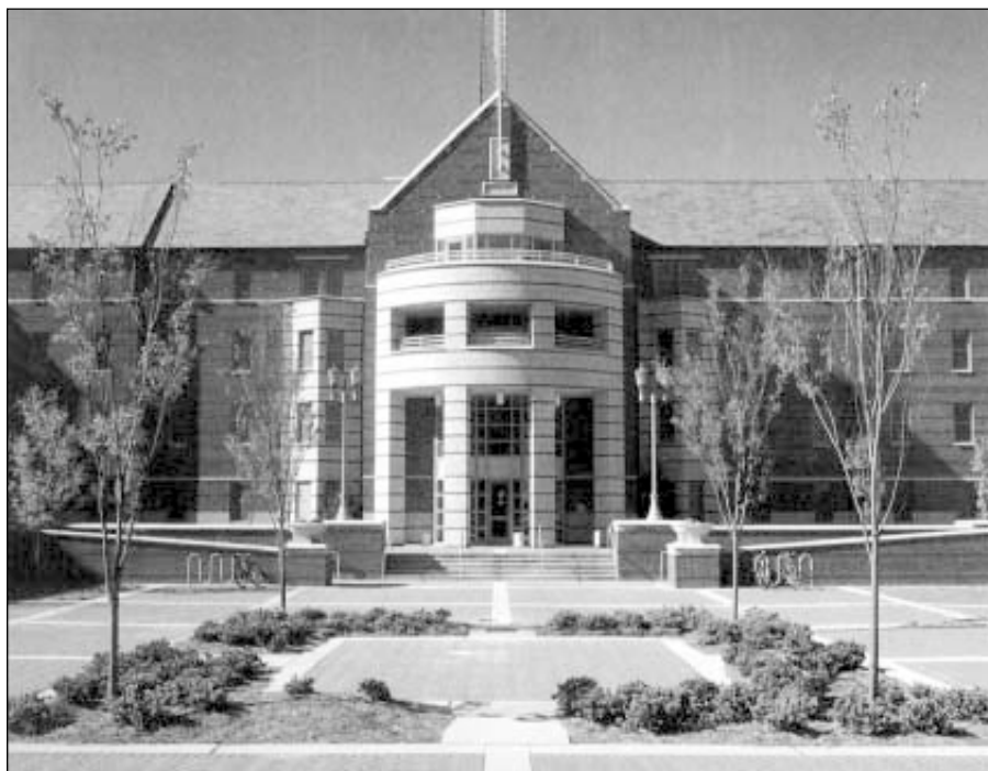
The system in place at the new Undergraduate Living Center on the campus of the Georgia Institute of Technology has been providing the center with humidity-controlled, temperature-neutral air using a dual-wheel, total-energy-recovery concept.
